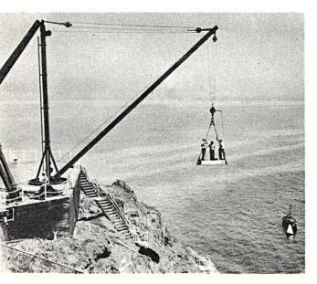
This "elevator" for the lighthouse keeper at Anacapa Island, off the coast of California, rises 180 feet from sea level to a loading platform at the edge of the cliff below the tower.
