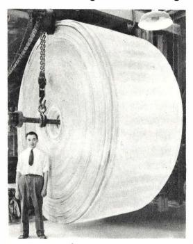
This conveyor belt, one of world's largest, weighs 11 tons.
