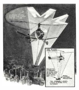
Hovering almost motionless in the air, this autogiro, equipped with magic lanterns, can present aerial advertisements at night by using the rotating blades as a screen. Inset—Side view, showing method which is used to project the message.
