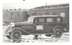
This built-in jack, mounted directly under the center of gravity, serves as a convenient turntable for this rail car. It is the only type of jack which can lift the entire car at once.
