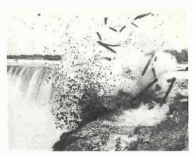
A charge of dynamite, weighted down by railroad ties gave Niagara Falls her latest face lifting operation. Water had so undermined the clift that it was a menace to sight-seers.
