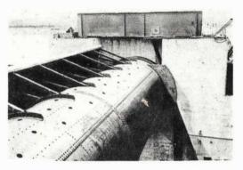
A view of the roller-gate dam at Canton, Mo. Just behind the steel gate is the concrete piece in which are installed 6 mammoth water heaters; these melt ice around dam in winter.
