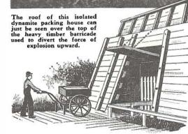
Drawing shows the rubber-tired carriage used to transport tanks of nitroglycerin from storage vat to the mixing house. Dynamite house doors always swing outward for instant exit.
