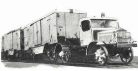
Through dual purpose trucks such as are shown above, the French State Railway system hopes to be able to furnish scheduled freight service to all communities now reached only by truck. At the left the lorry-train is shown mounted on flanged wheels for rail service, and on the right it is shown with pneumatic tires, ready for overland travel.
