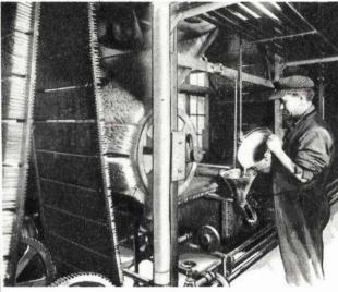
Pouring liquid chemicals into tipping machine. Note bristle-like matches on belt being carried through three compositions in which match heads are dipped to form the combustible crowns for striking.
