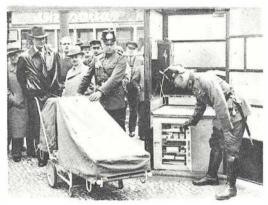
Fully supplied with all the equipment necessary to administer first aid, emergency stations like the one above have been established in telephone booths on Berlin's street corners. The wheeled stretcher folds into tiny compartment below telephone.
