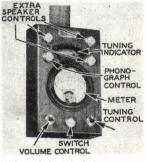
A view of the 7-inch long remote control box, showing instrument panel. It can be used anywhere.
