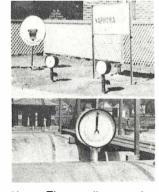
Above—These gasoline measuring gauges eliminate the need for poles in measuring the contents of underground tanks. Below—The gauge installed on a bulk tank.
